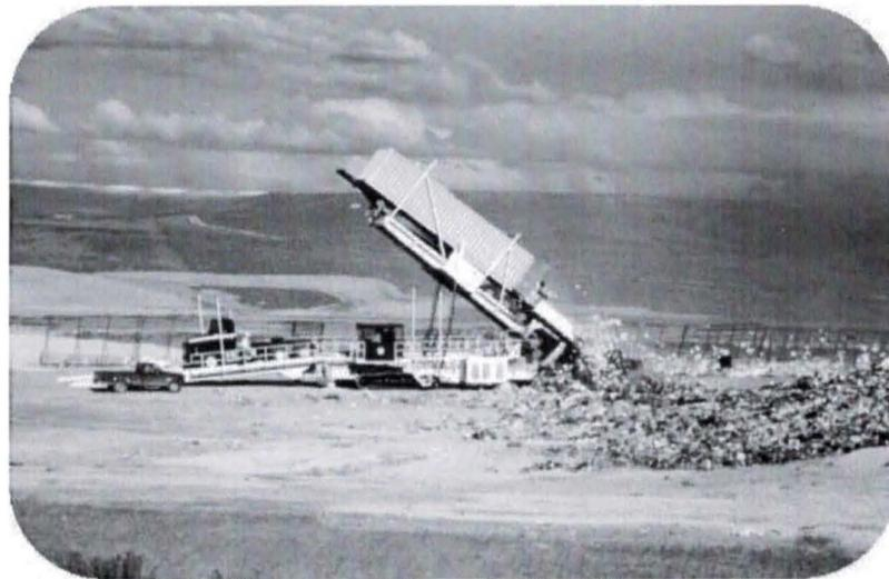
Figure 2-5. Tipping of a Waste Transfer Trailer at the Columbia Ridge Landfill
